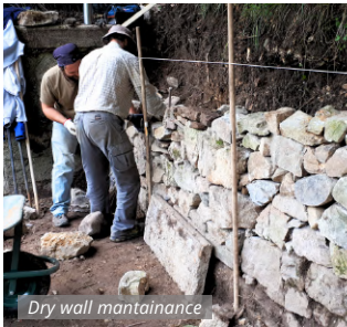
Dry wall maintenance
